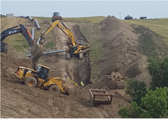
Storm Drain Infrastructure, Cherry Creek Community
