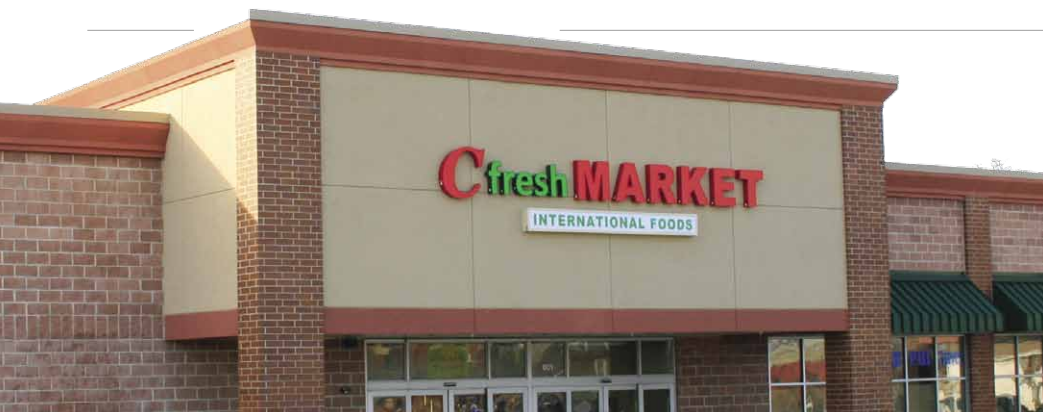
The C Fresh Market is the first full-service food retailer to operate in its Des Moines neighborhood in nearly a decade. Roughly one-third of the market's financing came from an HFFI-funded loan.
