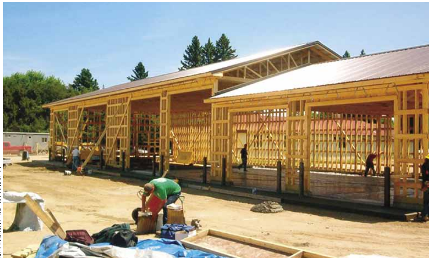
PHOTO COURTESY OF FRONTIER CONSTRUCTION A Frontier Construction project site. The company is one of many Native-owned contracting firms that have had difficulties in obtaining surety bonds.
