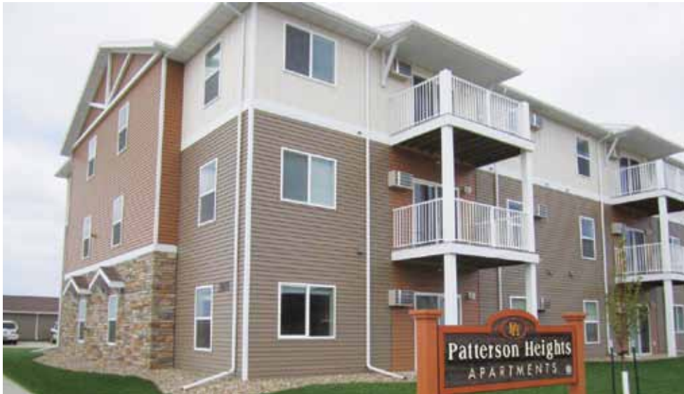
North Dakota Housing Incentive Fund (HIF) dollars helped Beyond Shelter, Inc., develop Patterson Heights, a 24-unit apartment complex in Dickinson, N.D. One-third of the building's units are set aside for law enforcement personnel.
