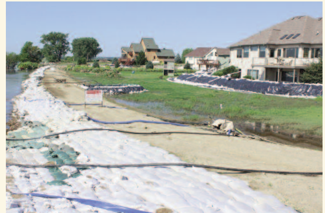
Multiple pump hoses carry groundwater over a dike in rural Union County, S.D.
