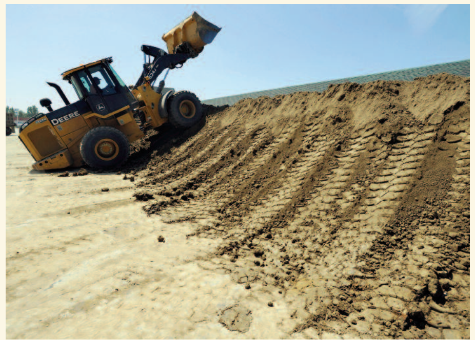
An earth mover packs down a dike as higher crest estimates of the Souris River were announced.
