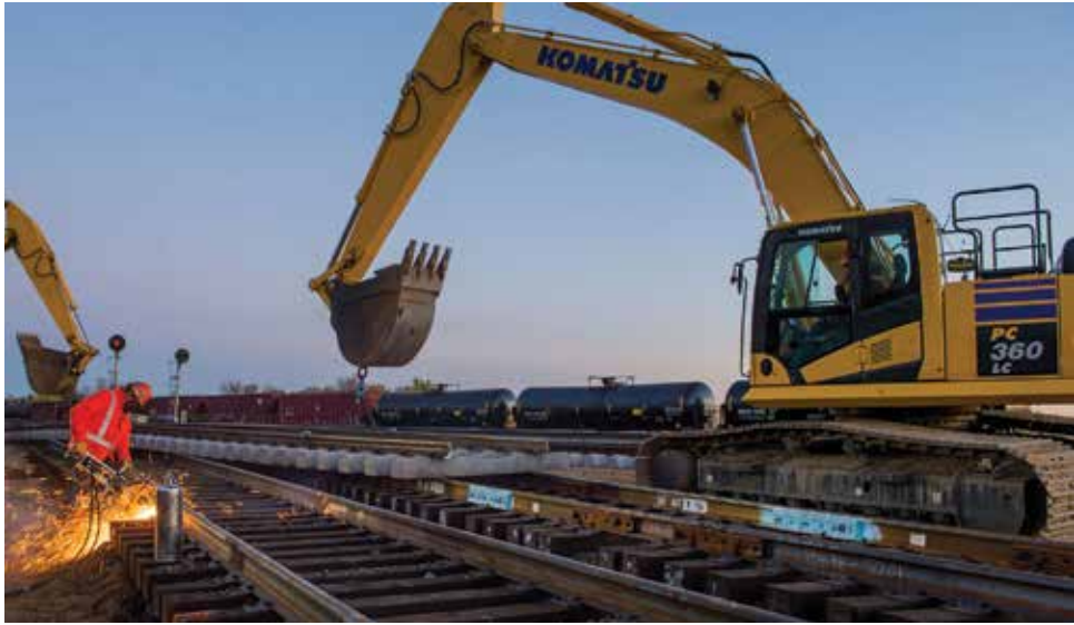
Constructing new BNSF track in North Dakota, where crude-by-rail traffic has surged.
