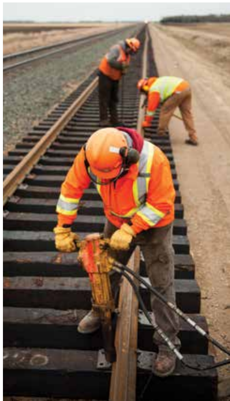
Canadian Pacific workers lay siding track near Wyndmere, N.D.
