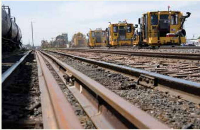
Track maintenance equipment stands ready at MRL's Laurel, Mont., yard.
