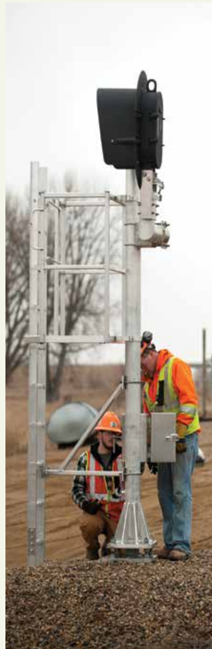
Workers installing CTC on a Canadian Pacific line in North Dakota.
