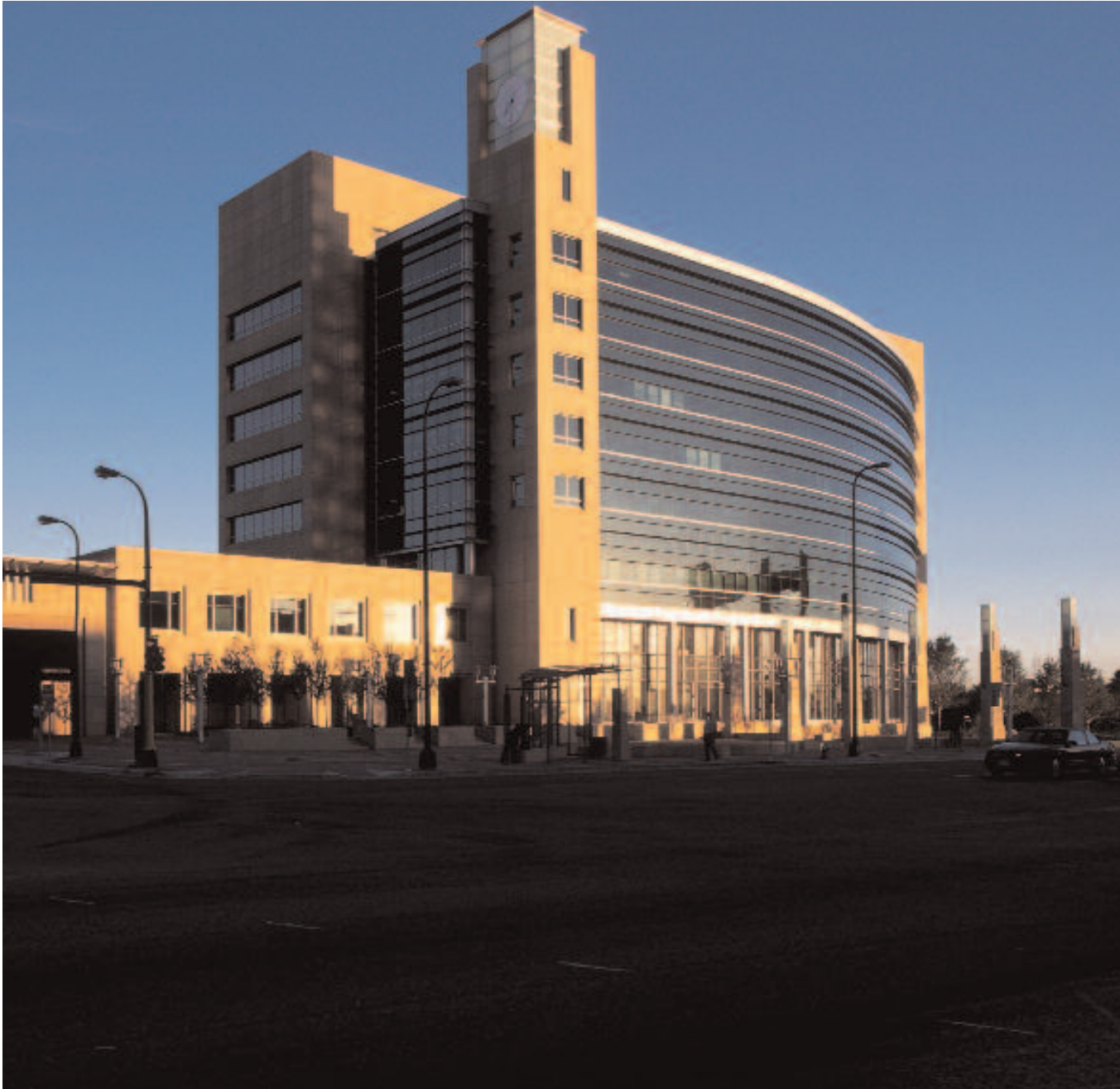
Federal Reserve Bank of Minneapolis
